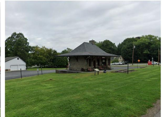
Rain gardens can be installed north of the building and in the turfgrass area east of the building to infiltrate stormwater draining from the parking lot. A preliminary soil assessment suggests that more soil testing would be required before determining the soil's suitability for green infrastructure.
