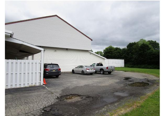
Porous pavement can be installed along the parking spots in the back lot of the building. The downspouts currently empty onto asphalt which is impervious and does not aid in infiltration. A preliminary soil assessment suggests that the soils have suitable drainage characteristics for green infrastructure.
